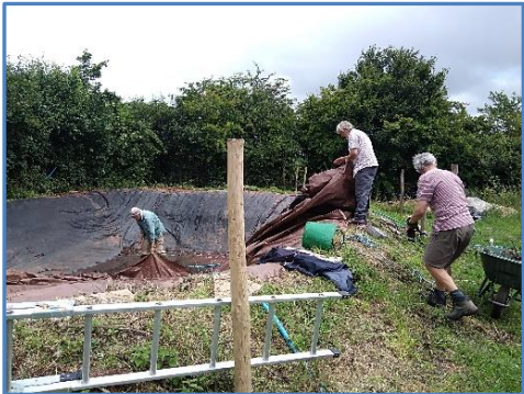
The Reservoir has been re-lined
