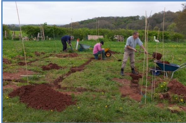
Digging shed foundation 2012
