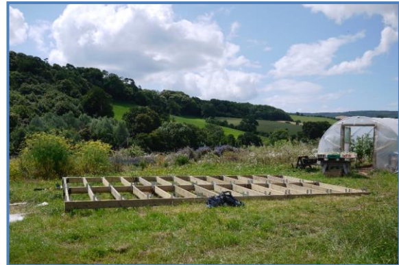
Shed floor joists 2012
