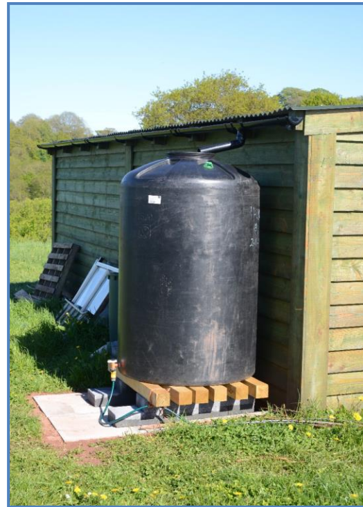
Shed water tank 2013
