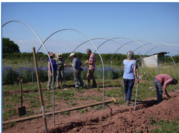
Building our first poly tunnel July 2011
